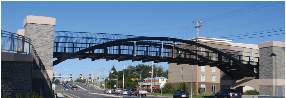
Pedestrian Bridge, Christiansburg
